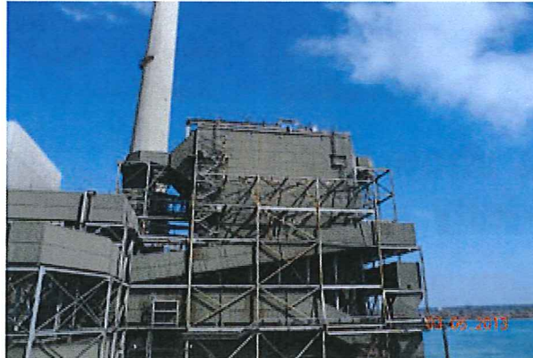
This St. Clair Power Plant photo shows the south side of the ESP on Unit 6. Photo supplied by David Nordstrand.
